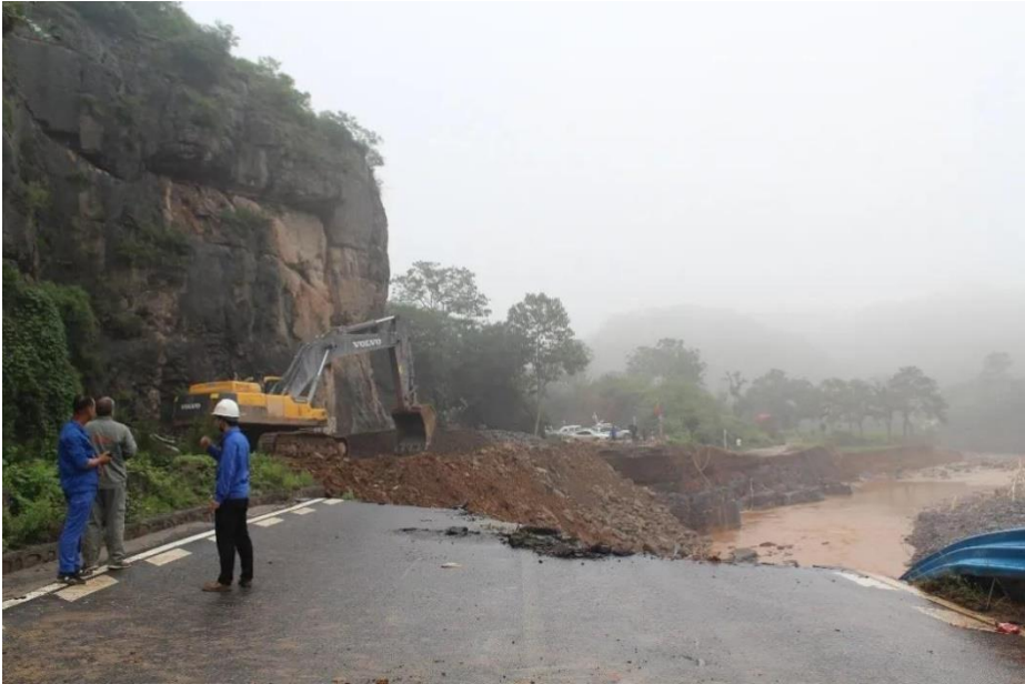
The Group Uses Excavators to Repair 234 Provincial Highway
