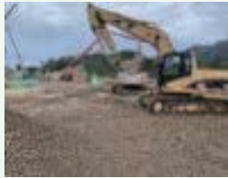
Used for roadbed cushion
