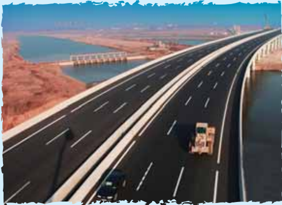
Tangshan Binhai Avenue Project
