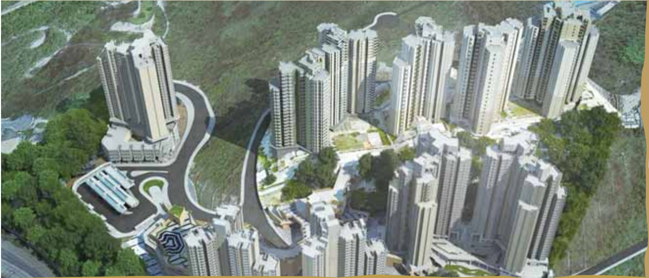
Construction of Public Rental Housing at Sha Tin Area 52 Phase 2
