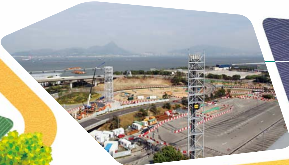
Project Name APM and BHS Tunnels on Existing Airport Island
