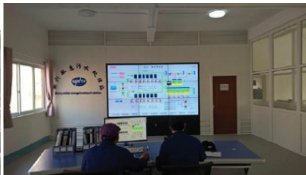
Water treatment laboratory
