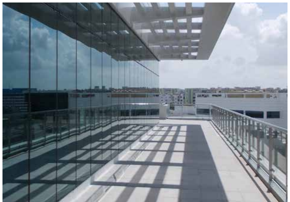
Double-glazed low-energy transparent glass for energy-saving
