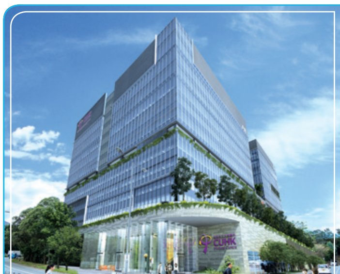
CUHK Medical Centre, Hong Kong
