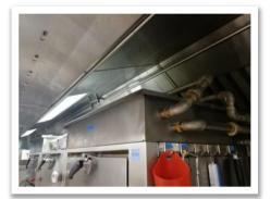
(Diagram: steam recovery equipment to generate hot water, make the best use of resources and energy)
