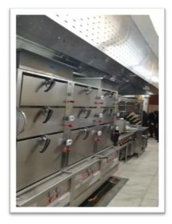
(clear steam cabinets switching time and separate switch for each steaming grid)
