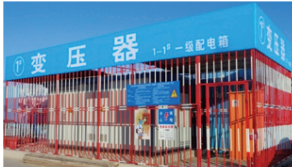
Protection for box transformer
