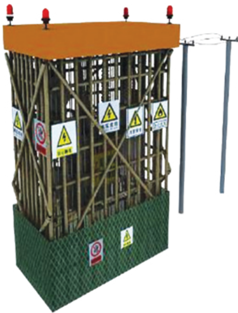
Protection for transformer
