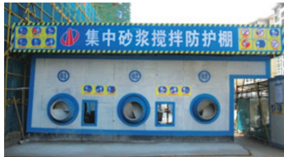
Setting up rain-proof and anti-smashing sheds
