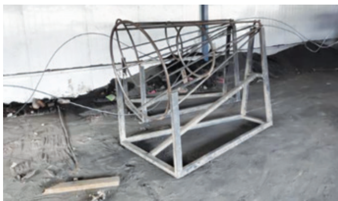
Protection for rebar straightening
