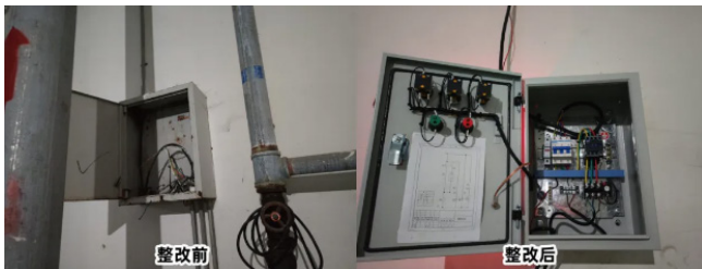
Rectification of sewage pump in underground garage 地下車庫排污泵整改
