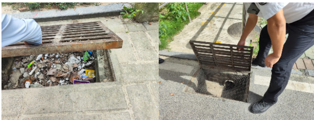
The rectification of road drainage outlet in the park 園區路面排水口整改前後
