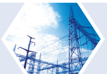
Power Remote Monitoring Solution
