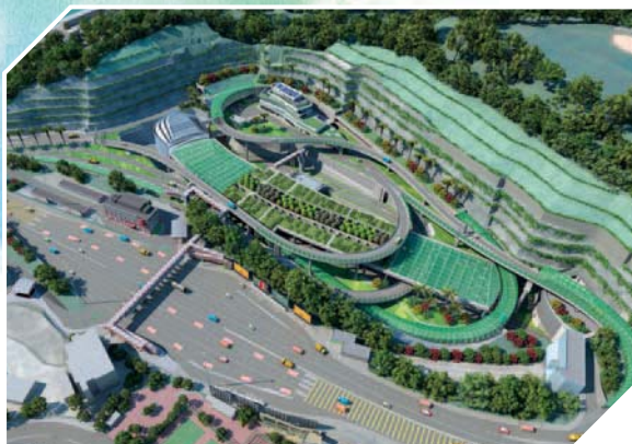
Tseung Kwan O — Lam Tin Tunnel
