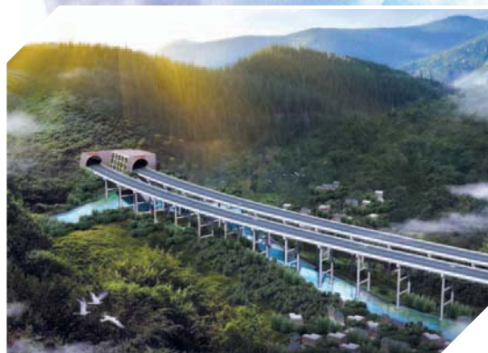
Highway PPP Project from Yinjiang, Guizhou Province to Xiushan, Chongqing
