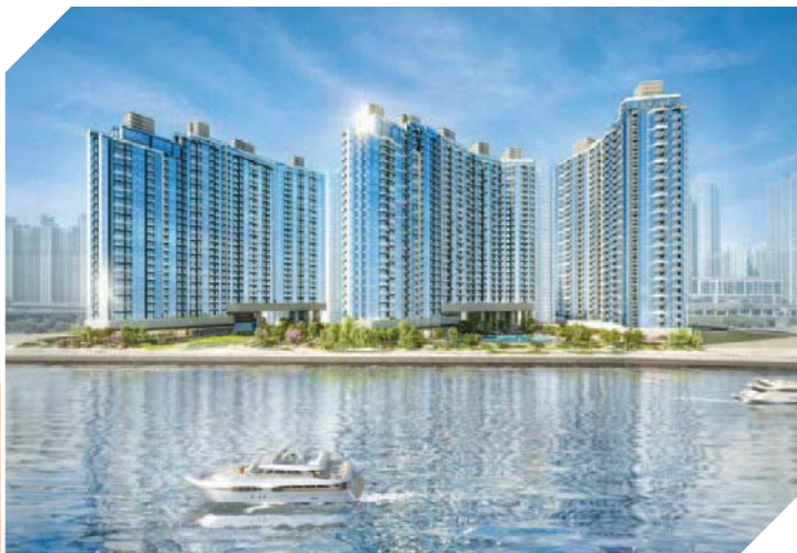
Residential Development at Hing Wah Street, Cheung Sha Wan
