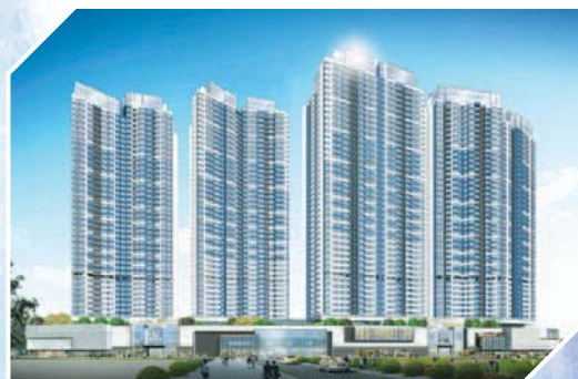
The Construction of the Residential and Commercial Development Project of Nova City Phase 5
