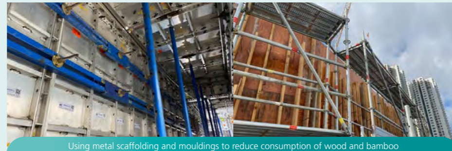
Using metal scaffolding and mouldings to reduce consumption of wood and bamboo
