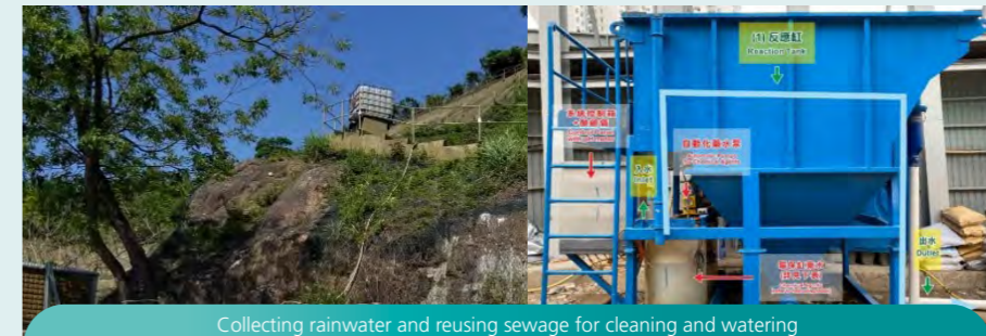
Collecting rainwater and reusing sewage for cleaning and watering
