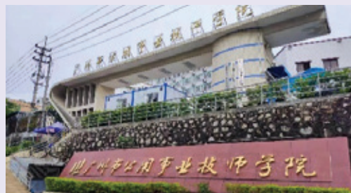
Guangzhou Public Utility Technician College
