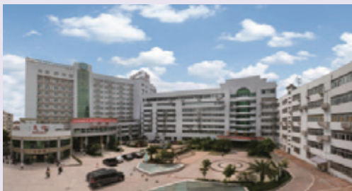
Yudu County People's Hospital
