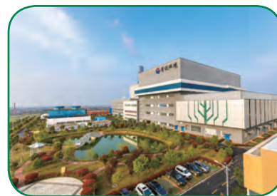
Nanchang Quanling Power Plant
