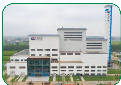
Xihua Collection and Transfer Project
