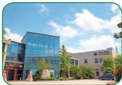
Hangzhou Anaerobic Treatment Project
